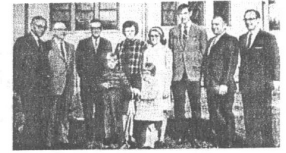
GROUNDBREAKING FOR 1968 ADDITION
